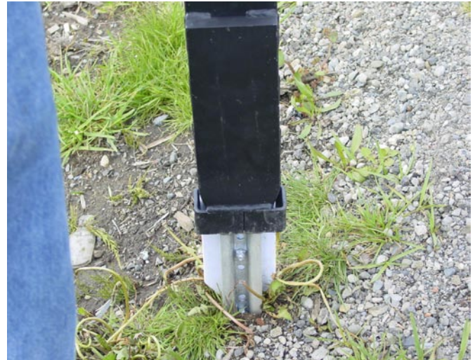
4. Repeat Process Until Anchor is at Least 2" (5cm) below ground.
