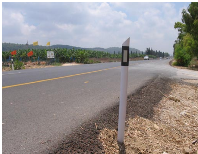
FG 500 Post Properly Installed
