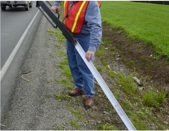
1. Place Delineator Post into Driver
